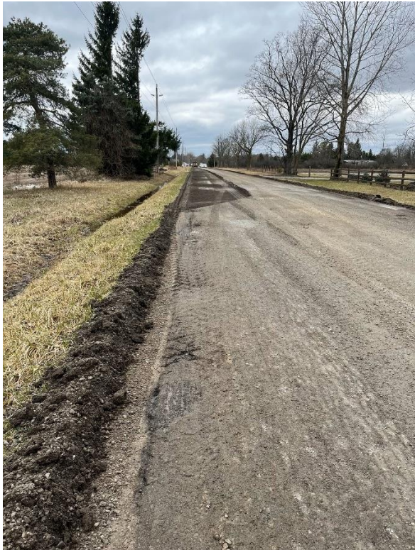
Foss Road Emergency Road Repairs
